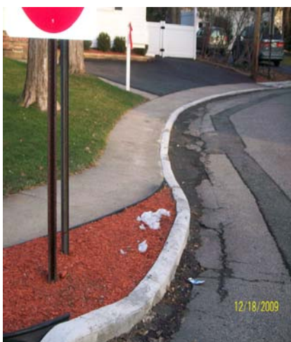
New Curb at Third Avenue
