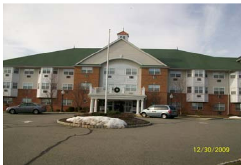
Pictured is Cook's Pond Senior Housing, located on Diamond Spring Road.
